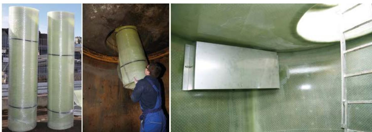
The flexibility, light weight and good processing qualities of GRP are particularly apparent when renovating separators, as the laminate can be rolled up like a carpet and therefore fed quite easily through the manhole of the tank.
