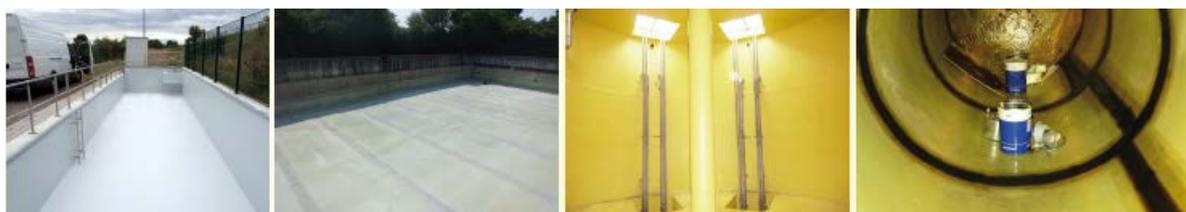
Whether a tank is large or small, open or cylindrical, GRP is suitable for the durable panelling of virtually any container.
