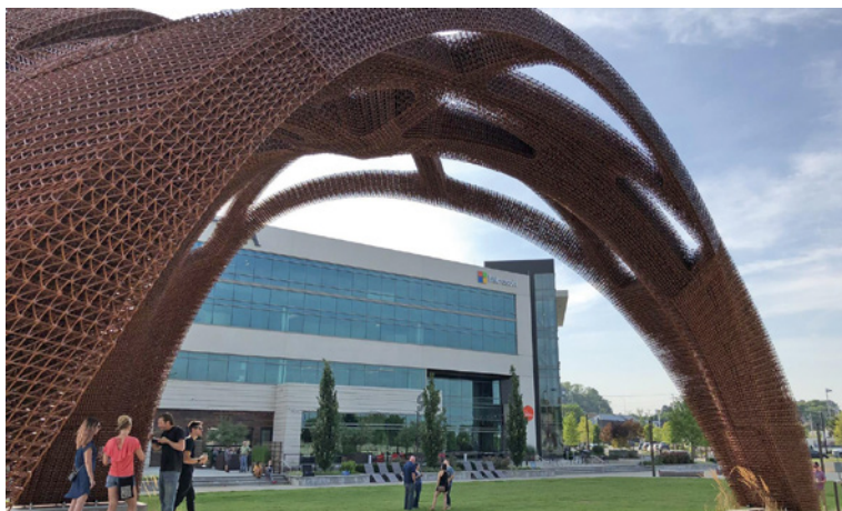
CFRP potential: Branch Technology has produced what is claimed to be the world's largest 3D printed structure
